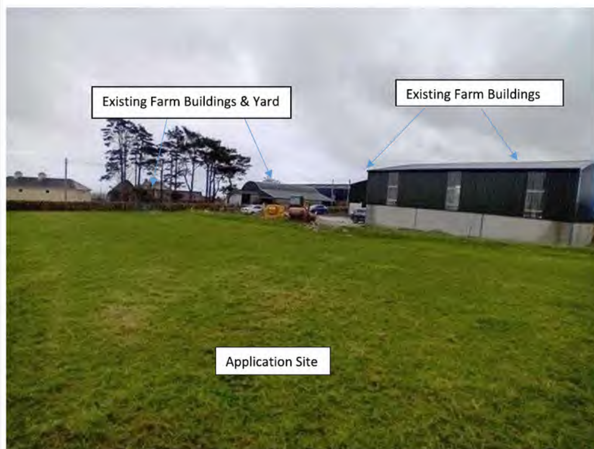
Figure 2- Application Site & Existing Farm Buildings
